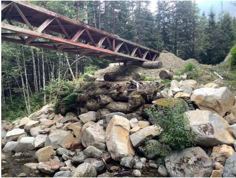
Right Bank Abutment when facing downstream
