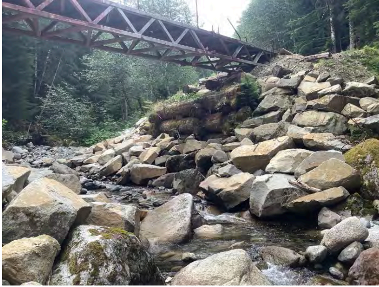
Left Bank Abutment when facing downstream
